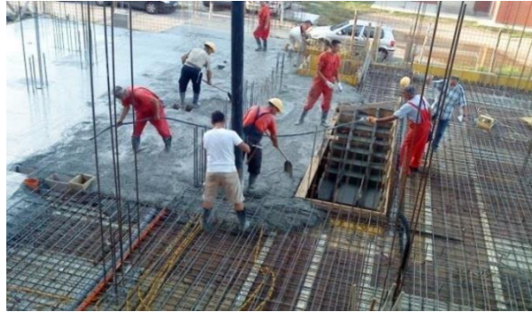
Figure 1 Concreting works for reinforcement slab
